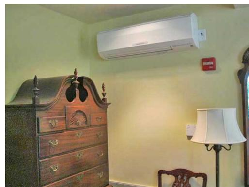
*Mini-split on the wall brings heat and cold from the heat pump into the room.*
