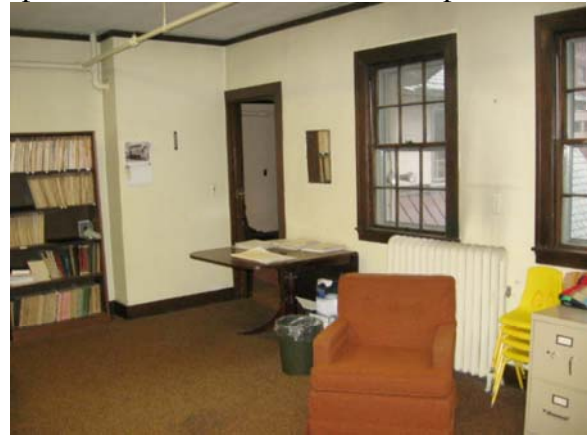
#10 — 2 nd floor music room is typical of smaller spaces with steam radiators. Install interior “storm” windows as low cost, high yield action.
