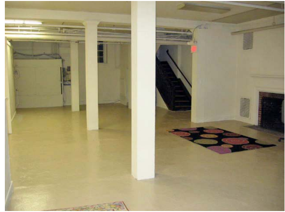
#8 — The basement space in the Parish House is to be rented. As the most used space, this is the first in line for energy upgrades. In-floor radiant is especially efficient in these locations. Lower ceilings to reduce CF of space needed to be heated.
