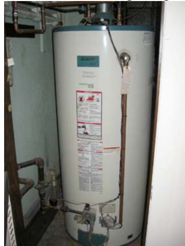
#4 (above) and #5 (below) — There are two DHW tanks — 40 gal electric and 75 gal gas. Efficiency is 65%±. Replace with one in-direct fired tank served by an efficient (93%) gas-fired boiler. This is part of a phased program of conversion to more efficient hydronic heating using high efficiency boilers, contemporary controls and zones matching use patterns.
