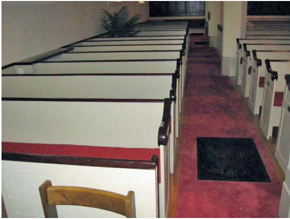
#5 — The sanctuary has steam radiation, both wall and via in-floor convection radiation with return air ducts.
