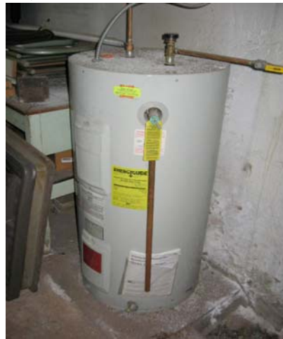
#4 (above) and #5 (below) — There are two DHW tanks — 40 gal electric and 75 gal gas. Efficiency is 65%±. Replace with one in-direct fired tank served by an efficient (93%) gas-fired boiler. This is part of a phased program of conversion to more efficient hydronic heating using high efficiency boilers, contemporary controls and zones matching use patterns.
