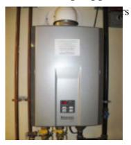
Standard domestic hot water ("DHW") vertical tanks are not very efficient (65±%) even when DHW is needed; they are 0% efficient when DHW is not needed. (Heating water that you are not going to use is by definition wasteful and expensive! You don't keep the tea kettle heating on the stove for a morning cup of tea!). On-demand water heaters are 84>95% efficient and they use energy only when generating DHW.
