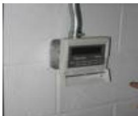
In addition to installing a new heat pump, a **programmable thermostat** was installed to control the system. This installation solved many of the problems experienced with the manual thermostat, including time on-and-off. (See photo at left.)
