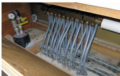
The Sanctuary was cleared, with the placement of pews carefully plotted for replacement without penetrating any new radiation piping. Old concrete was removed. New “plastic” piping installed with distribution to multiple loops through two
