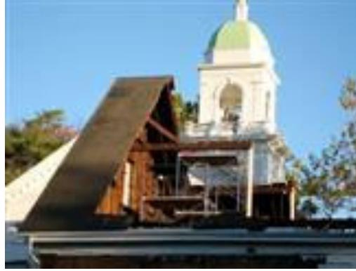
The roof over the old Parish Hall no longer met building code requirements for structural loads from snow. The new roof has a lower pitch, giving the historic Sanctuary more prominence. Roof has 12" blown fiberglass insulation.
