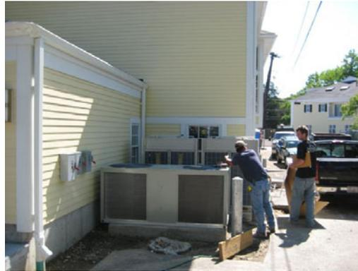
The high-efficiency HVAC (Heating, Ventilating, and Air Conditioning) system is connected to an Energy Management System (EMS) that allows the user to modify the heating schedule remotely via the Internet.
