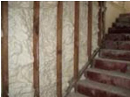
4" Icynene foam insulation was used in basement walls. All other parts of the church are insulated with either 6" or 12" blown fiberglass or cellulose fiber. Insulation ensures minimal thermal exchange between the building air and the outdoors.
