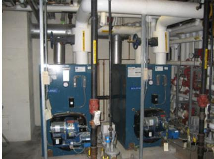
Temple Beth Shalom in Needham has made efforts in recent years to reduce energy bills and carbon footprint. In 2003, Beth Shalom switched from a low efficiency oil furnace to two gas-fired hydronic boilers that have 88% efficiency. (See photo at left.) At \$1.60 per gallon of oil compared to \$1.30 per therm, the new Burnham systems save the Temple \$3-\$4,000 every year.
