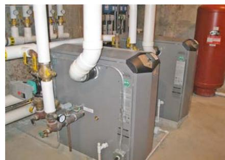
95±% efficient gas-fired condensing mode hydronic boilers, shown at right.
