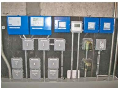
New controls and thermostats were installed. Heating zones were increased from 4 to 11. Domestic hot water (DHW) generation was converted to an in-direct fired storage tank using the high efficiency boilers. A computer-based Energy Management System (EMS) was incorporated for
